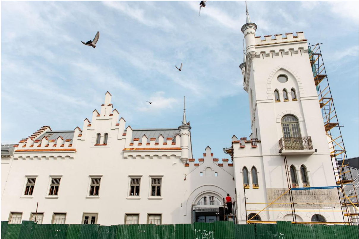
Factory after revitalization. Photo by Bohdan Yemets
